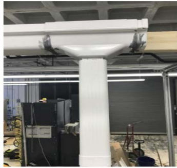
Fig. 1. Collected rainwater transfer device
